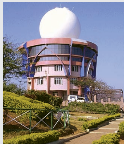
Doppler weather radar installation at Visakhapatnam
